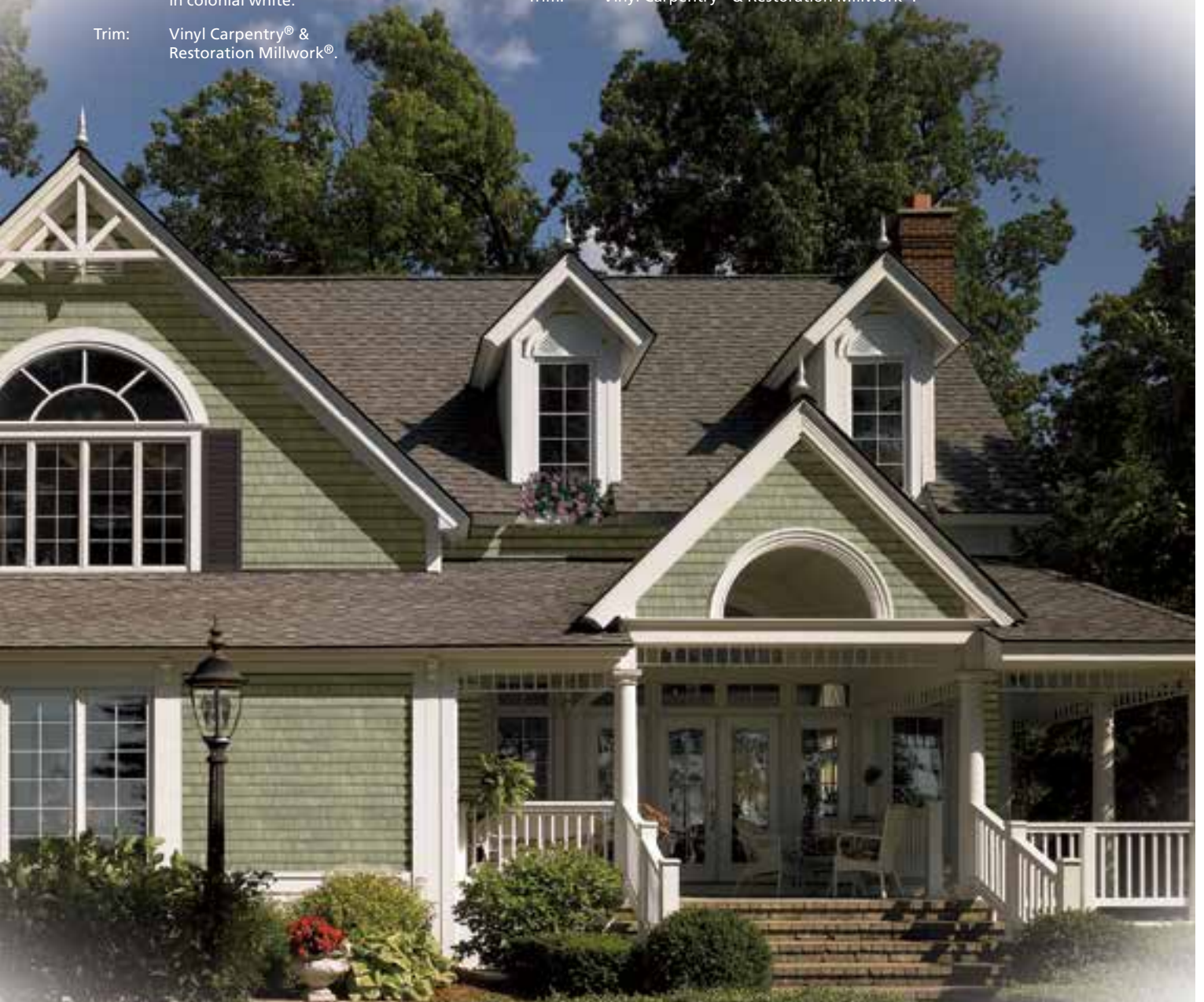
Siding: Triple 5" Straight Edge Perfection Shingles in cypress. Trim: Vinyl Carpentry® & Restoration Millwork®.
