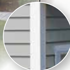
Restoration Millwork One-Piece Corner with InvisiGrip Hidden Fastening System
